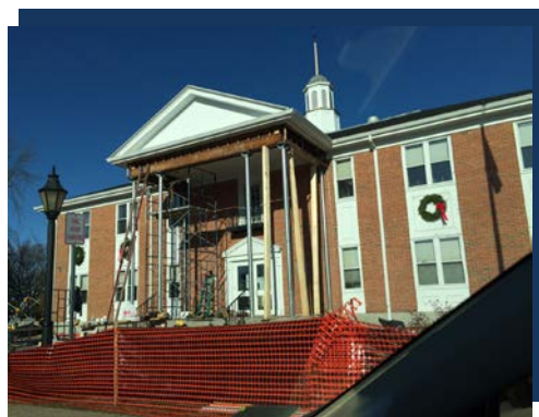
Main Town Hall renovation on deteriorating columns
