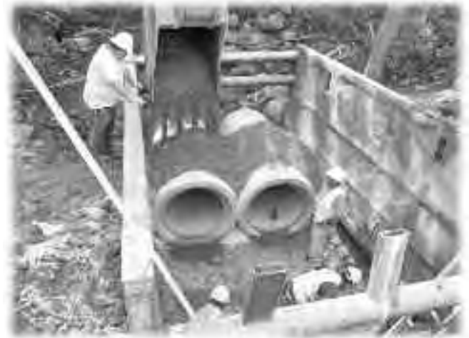
New Reinforced Concrete Pipe – Ray Ave Culvert
