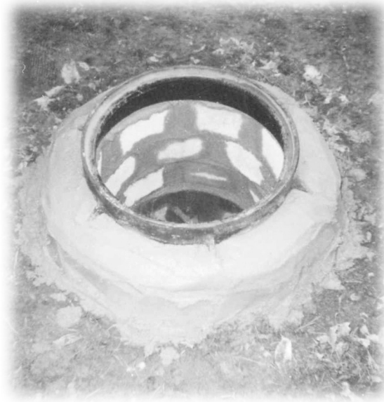
Repaired Sewer Manhole to prevent Inflow
