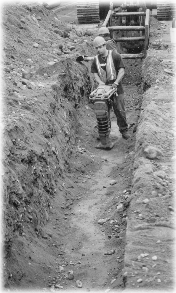
Water Main Trench Backfill and Compaction
